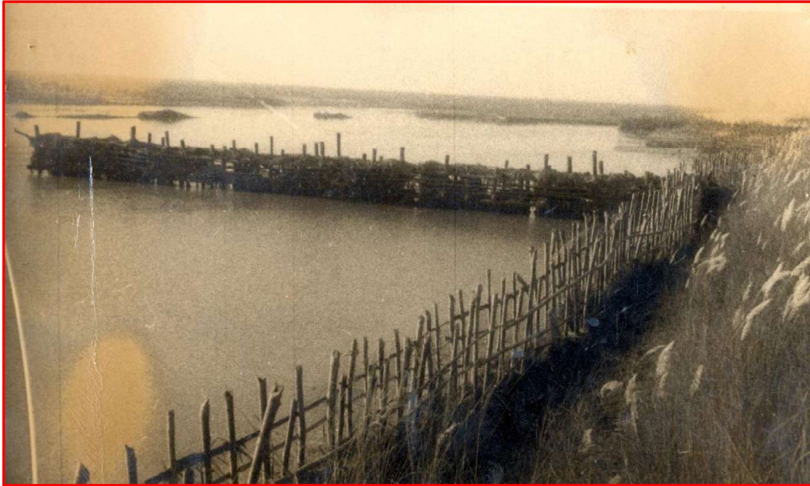
Bamboo screen and permeable spur
