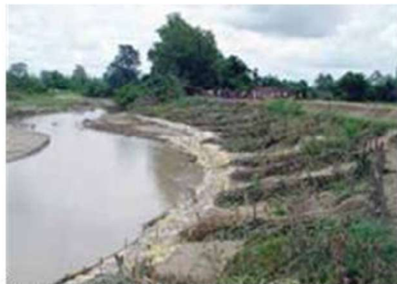
Figure 3. Low cost spur made of tree trunks and branches
