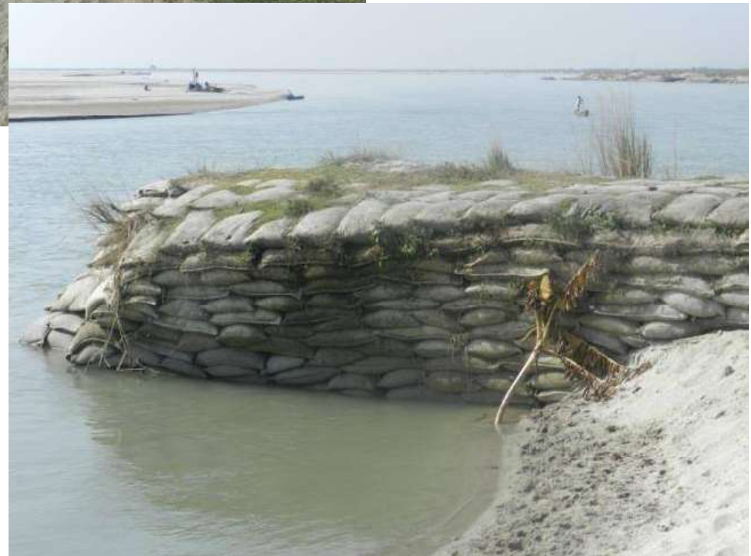
Flow diversion using studs immediately d/s of barrage
