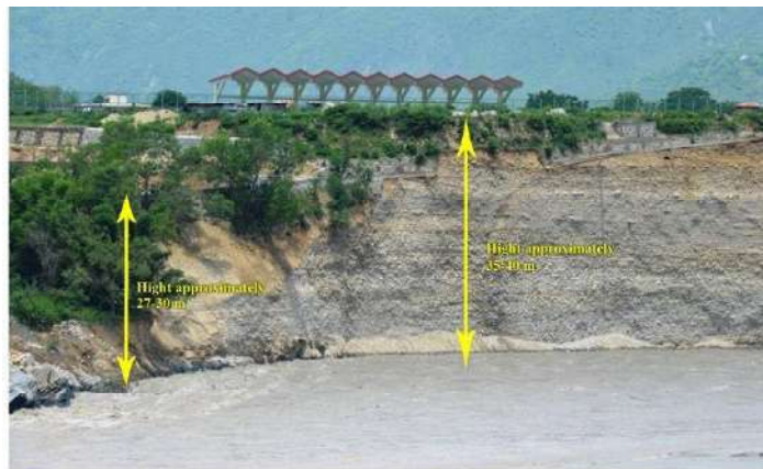
Photograph showing vertical profile of the affected site from river bed
