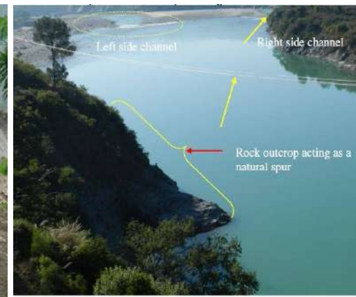
Photo 2: Rock outcrop at upstream left bank of erosion site.
