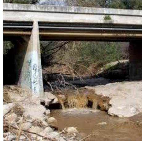
Figure 2.4 Bank erosion just downstream (Geomorphologic Factors affecting the scour depth)
