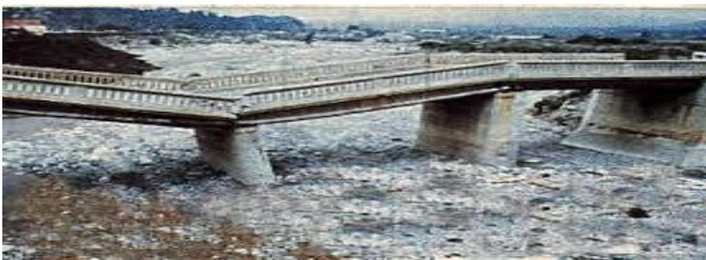
Figure 2.6 Bed sediment factors (causing bridge failure)
