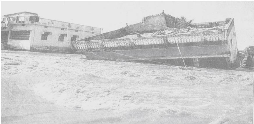
Fig. 1. Foundation failure due to scouring of ground at Begusarai, Distt. Kushinagar
