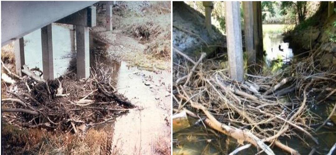
Figure 2.5 Floating debris accumulation at the bridge piers (Flood flow transport factors)
