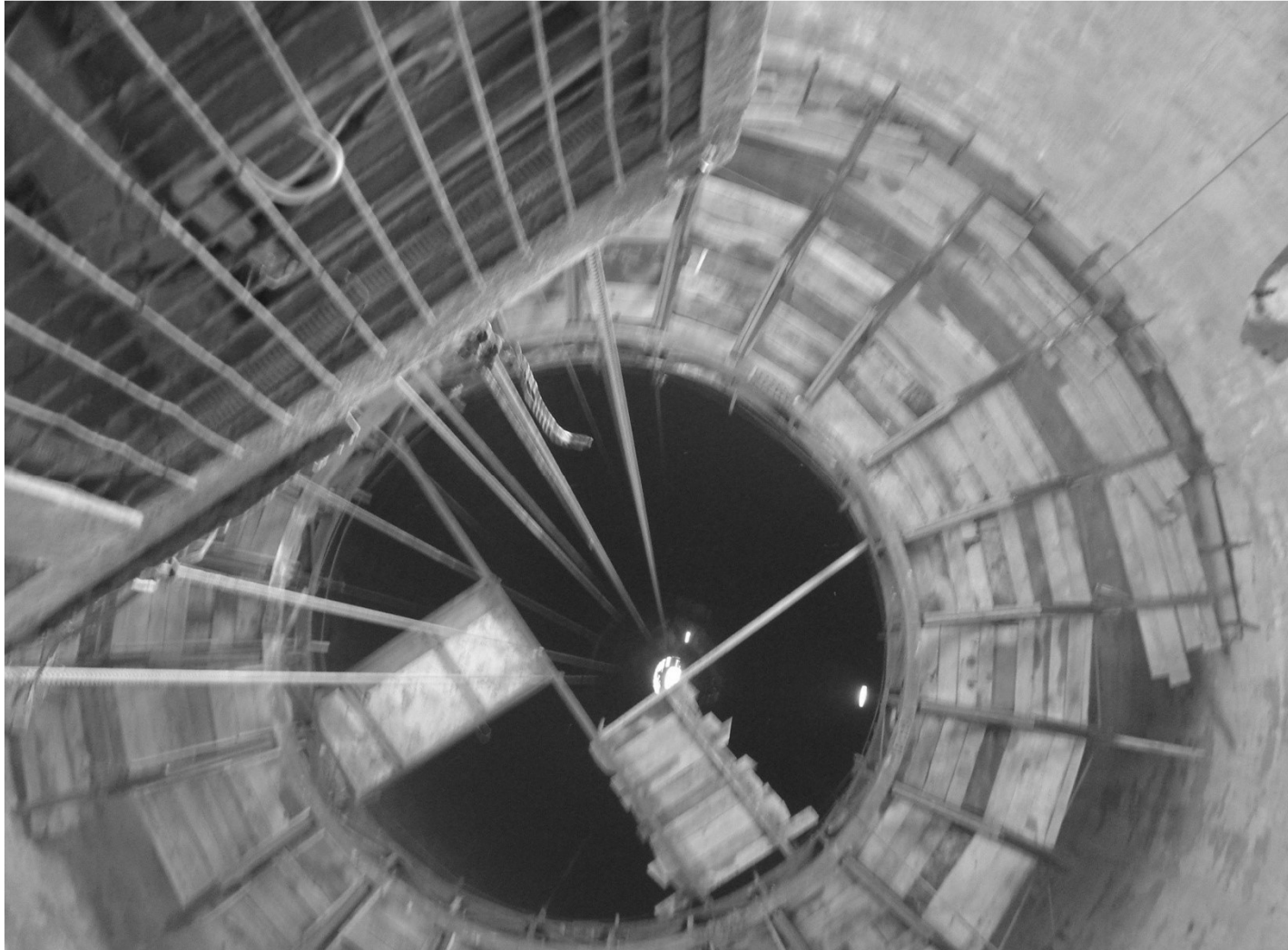
Chimney Under Construction
