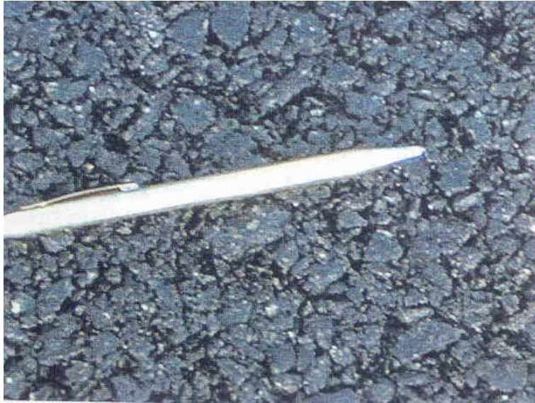
Freshly Laid BC layer
