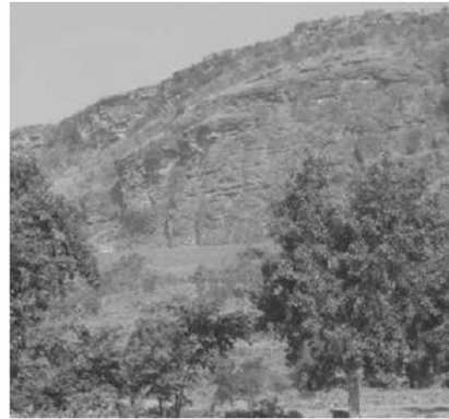
natural rock slope
