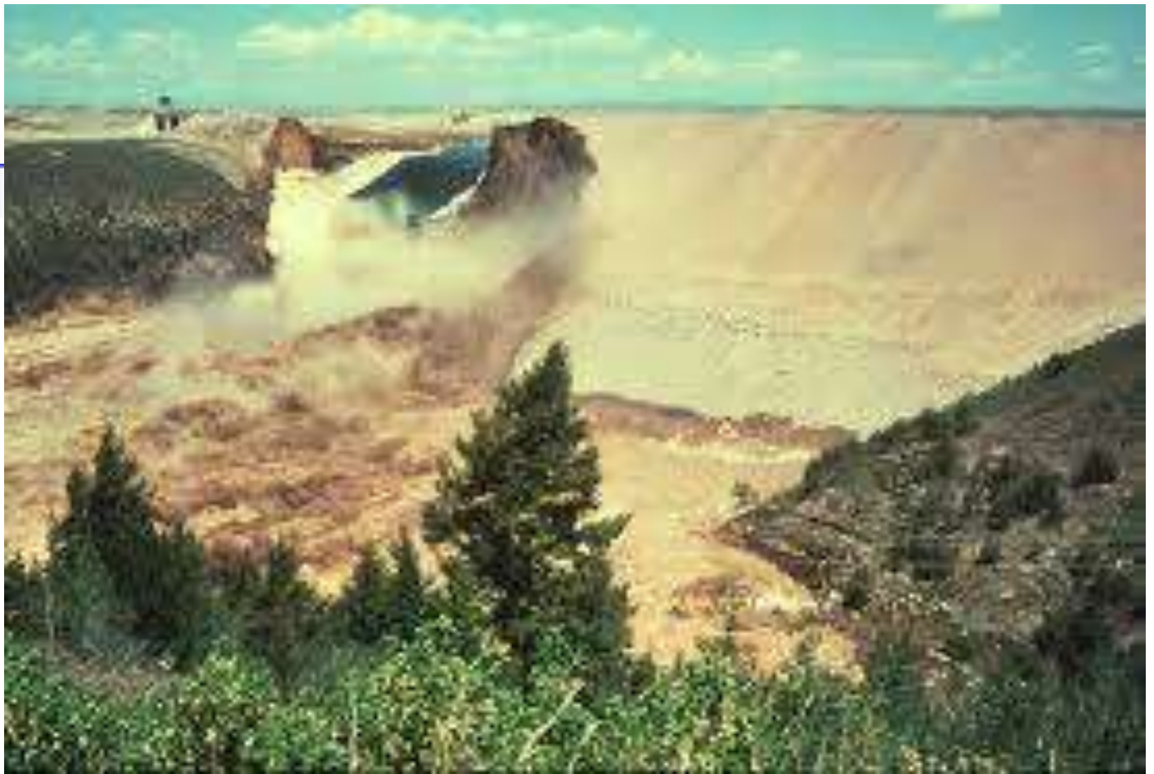
Failure of Teton dam, Idaho, USA
